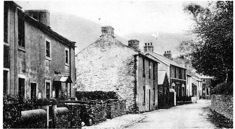
High Lorton street, soon after 1891, showing the old block at the entrance to Smithy Fold
