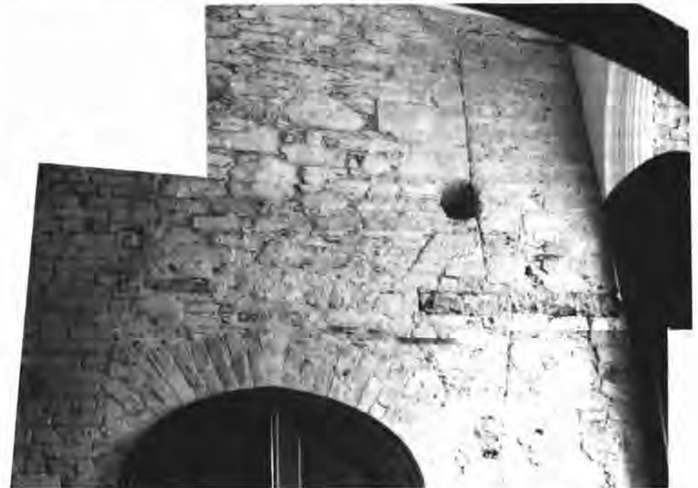
Photograph Nr. 1 - A montage showing the baptistry wall with the various modifications made to it, with possible evidence of a stairway, long since removed, into a lower chamber in the tower.
