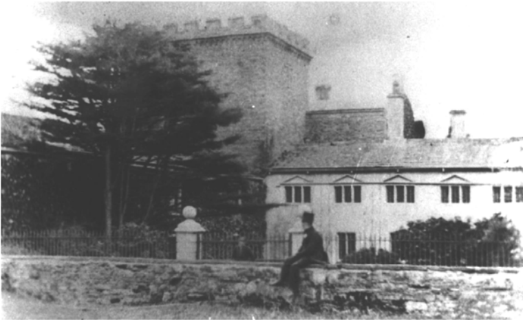
Figure 2. 1880s. Hall-range east facade of 1663. Before conversion by AJS Dixon, probably seated on wall. Viewed from Church Field showing gated entrance to courtyard, folly tower probably by George Lucock Bragg c. 1840, south wing intact. North, stables, wing out of shot. Photograph probably for AJS Dixon.
