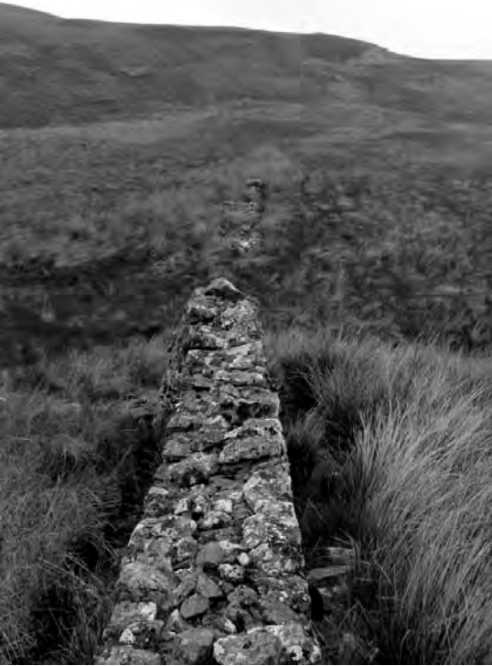
The dam looking west
