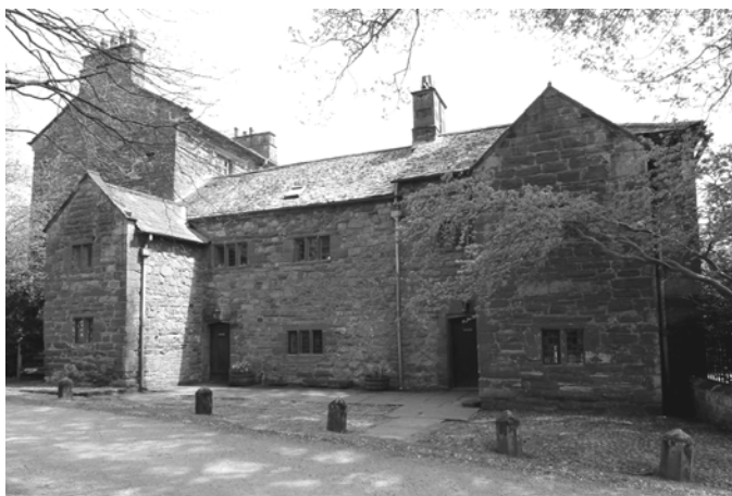
The C16th façade – photo Derek Denman
