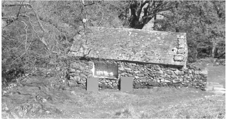
Figure 1. Borrowdale Mill – an example of a simple, manorial mill serving a Lakeland valley community. (Converted for residential purposes in 1936, it retains its original character, complete with overshot waterwheel. The elevated leat is visible on the left of the picture; a kiln was incorporated on the far side of the building when the storm-damaged mill was repaired in 1797).
