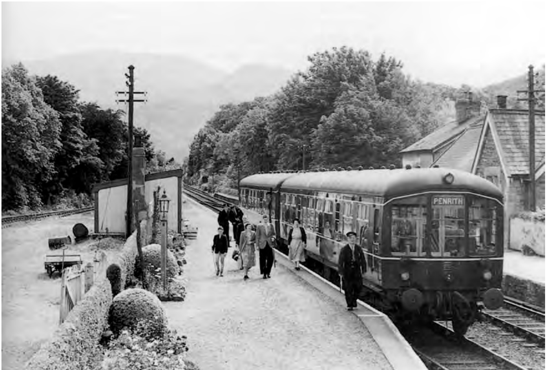
Bassenthwaite Lake station in the 1950s, images from Robert Western, The CK&PR
