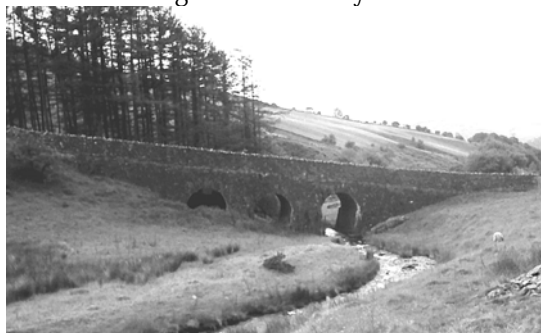
New Bridge from Spout Beck
