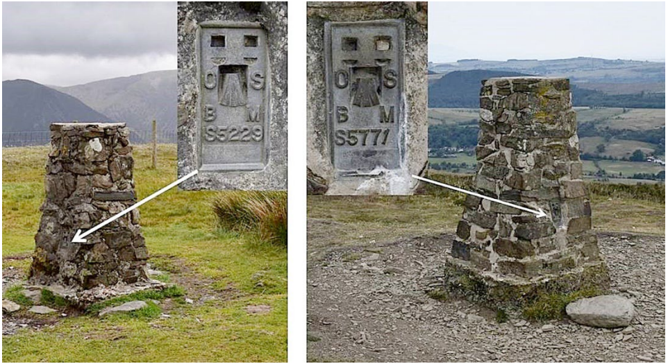
Figure 4. Triangulation pillars with S-series flush brackets on Fellbarrow (left) and Ling Fell (right). The pillars were constructed in the 1950s. Adjacent to the spider are three brass loops by which that equipment can be secured by cords.
