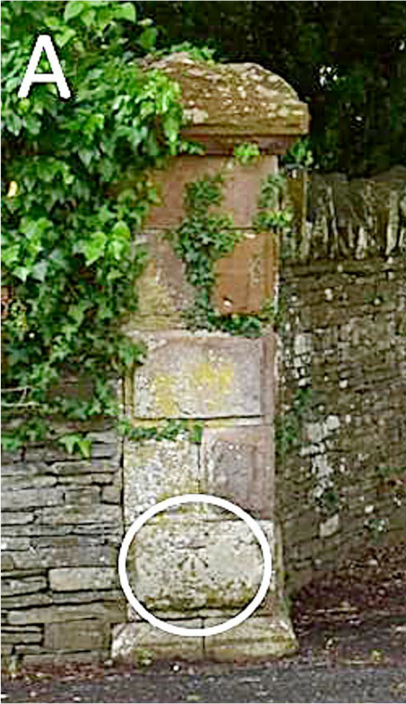
Figure 2. Selection of cut bench-marks (aka crow's feet) in the Lorton and Loweswater area.
