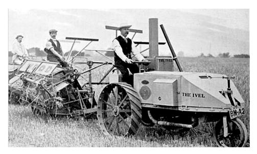
Figure 10. An Ivel Agricultural Motor pulling two reaper binders circa 1910.
