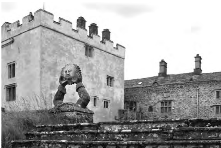
The pele tower and house front at Isel Hall, with the Lawson arms in foreground
